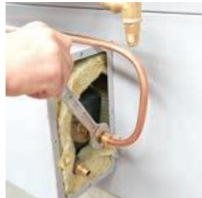
Fig. 6.3 Loosen the water input tube.
