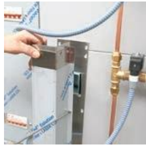
Fig. 6.1 Loosen the back steam output.
