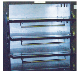
Adjustable Dampers at each deck
