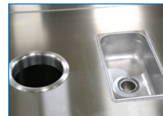
Liquid disposal and waste chute
